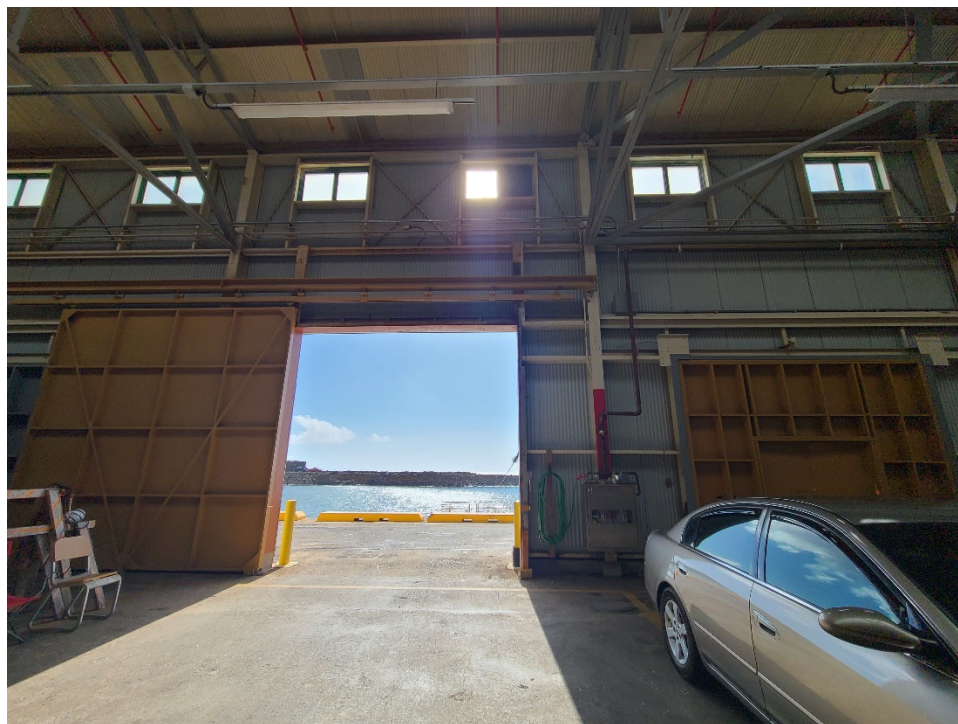
Photo 2: Typical Windows and Door Heads/Jambs/Guides
