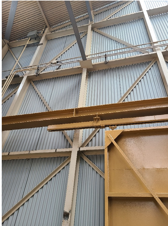
Photo 1: Typical Wall Section
